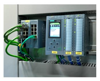
ACE also implemented the SCALANCE XB216 switch via a S7-1515-2 PN ensuring real-time communication across the network and with a separate CPU 1512SP F-1 PN for the safety of the production line.
